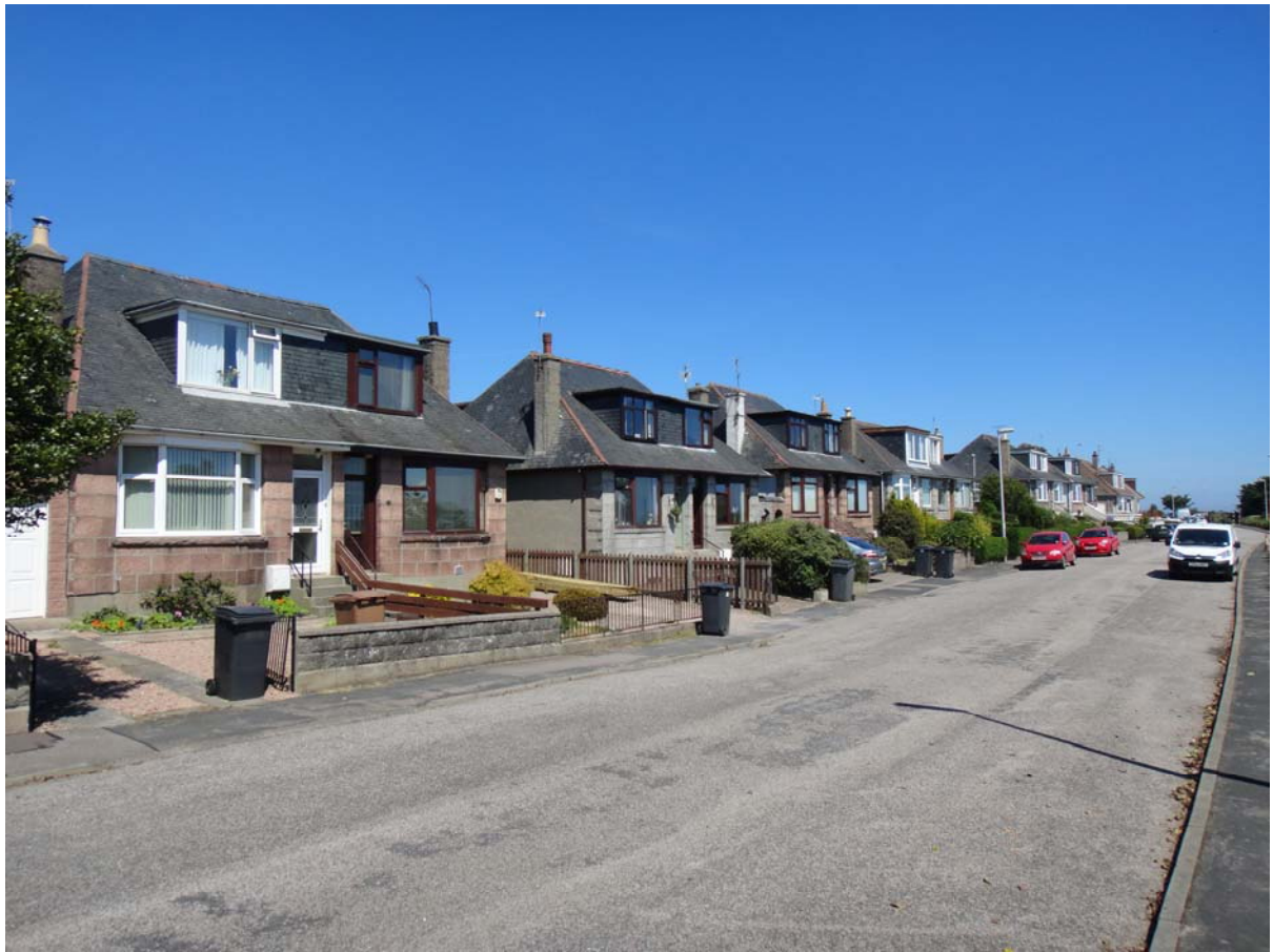
Front box dormers positioned in line with neighbouring traditional properties, Donmouth Road
