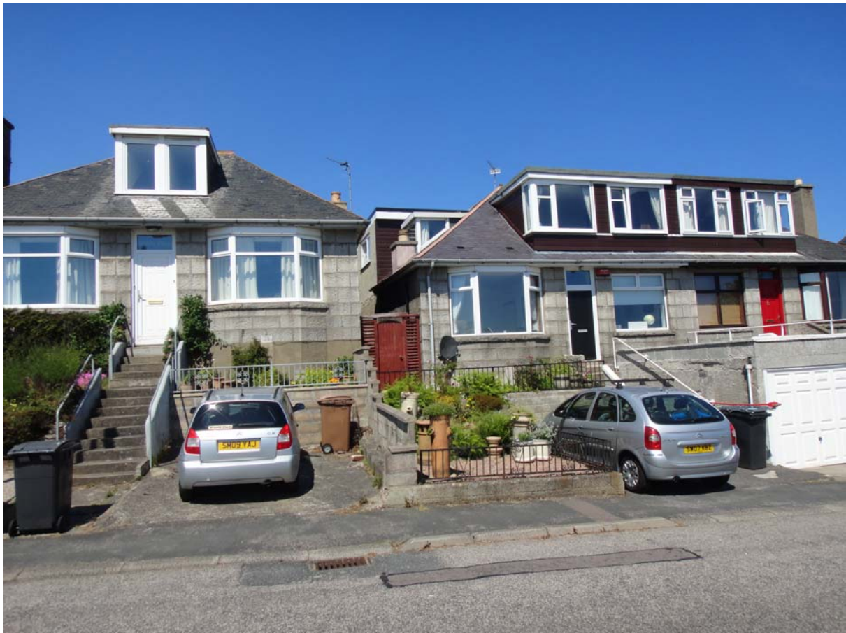
Front box dormers positioned on wall head, Donmouth Road
